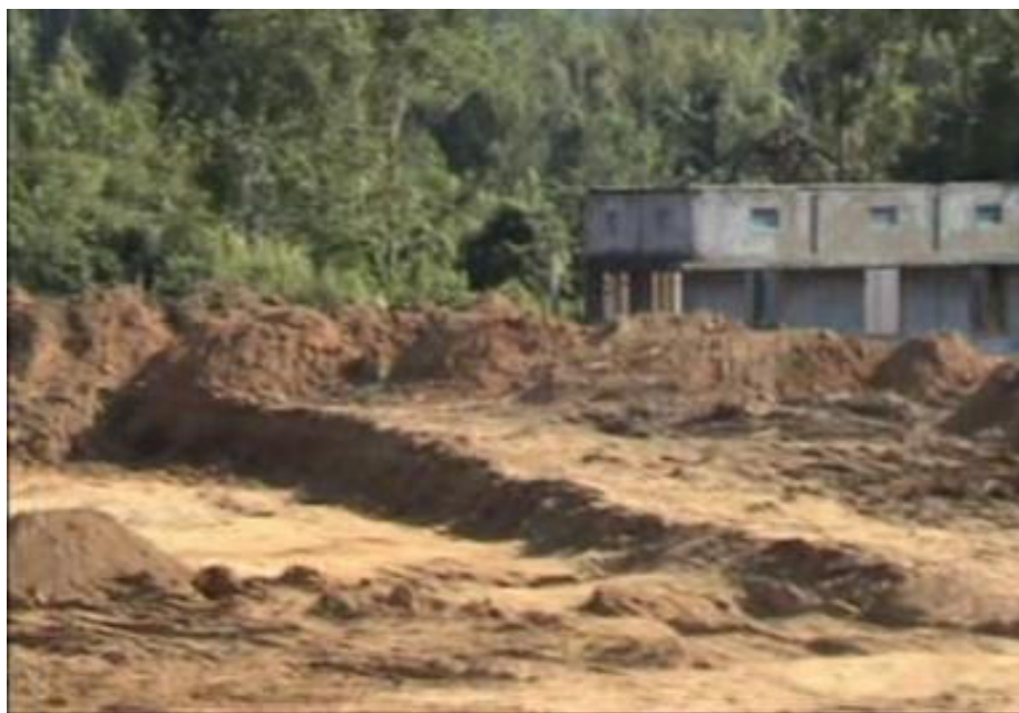
A demolished house with a barren land which cannot be inhabited by the villagers after 2003 ethnic conflict in a village of DimaHasao district.
