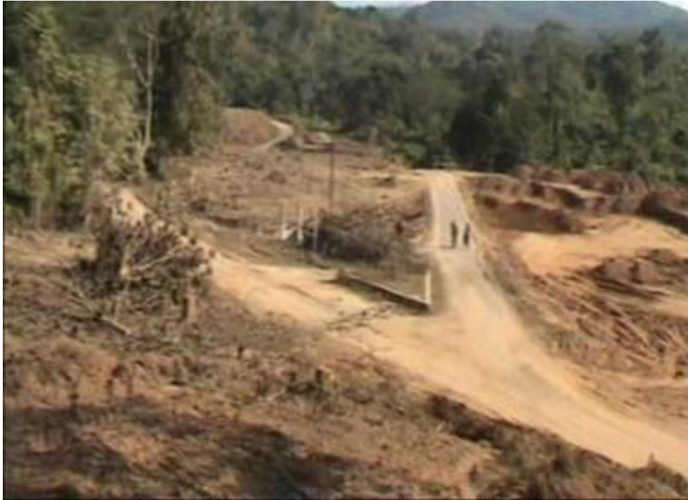
A village which was demolished in 2003 ethnic conflict has been converted into a National Highway.
