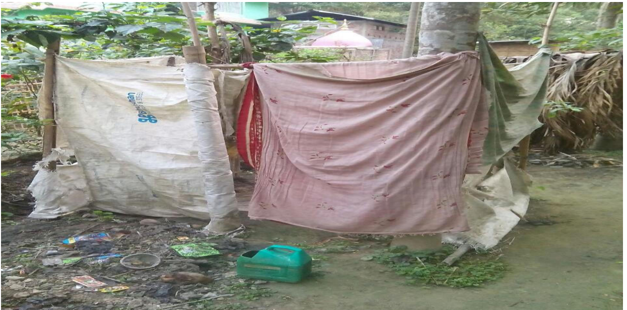
Picture X: View of Unhygienic Pit Latrine (Kuchha Latrine) in the Slum Area
