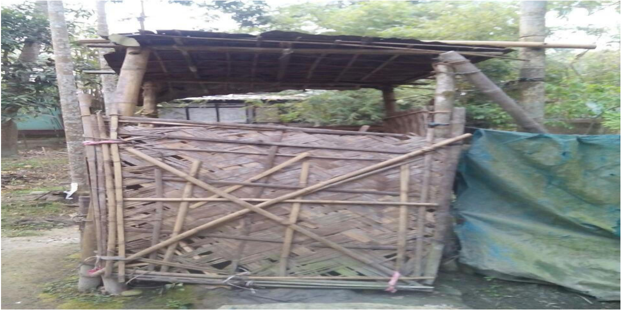
Picture IX : View of Unhygienic Pit Latrine (Kuchha Latrine) in the Slum Area
