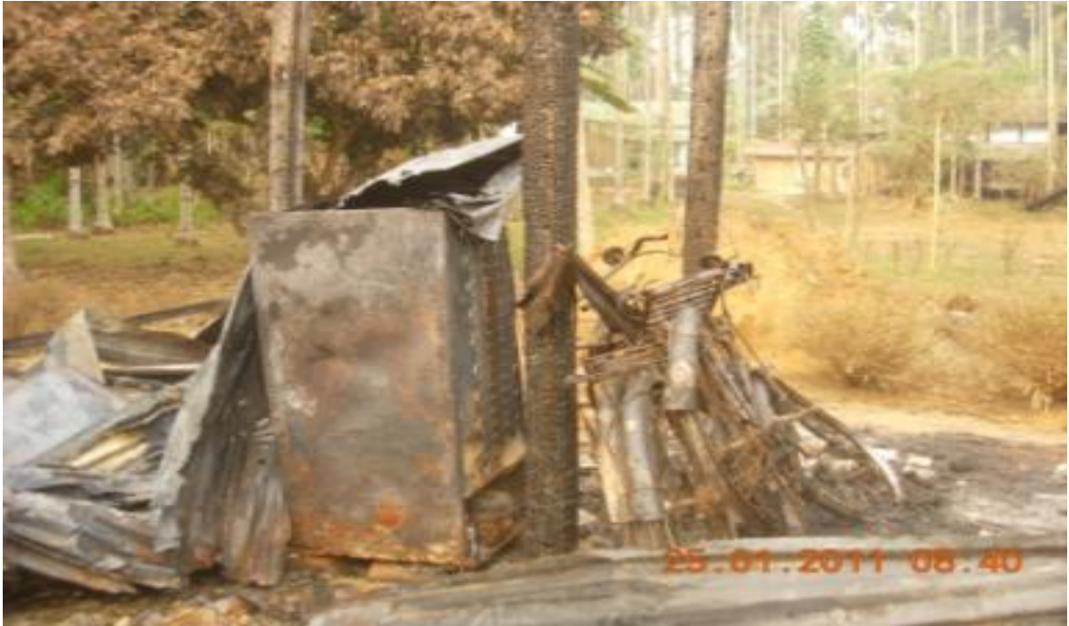
FIGURE 3: Household Properties Vandalize and Looted
