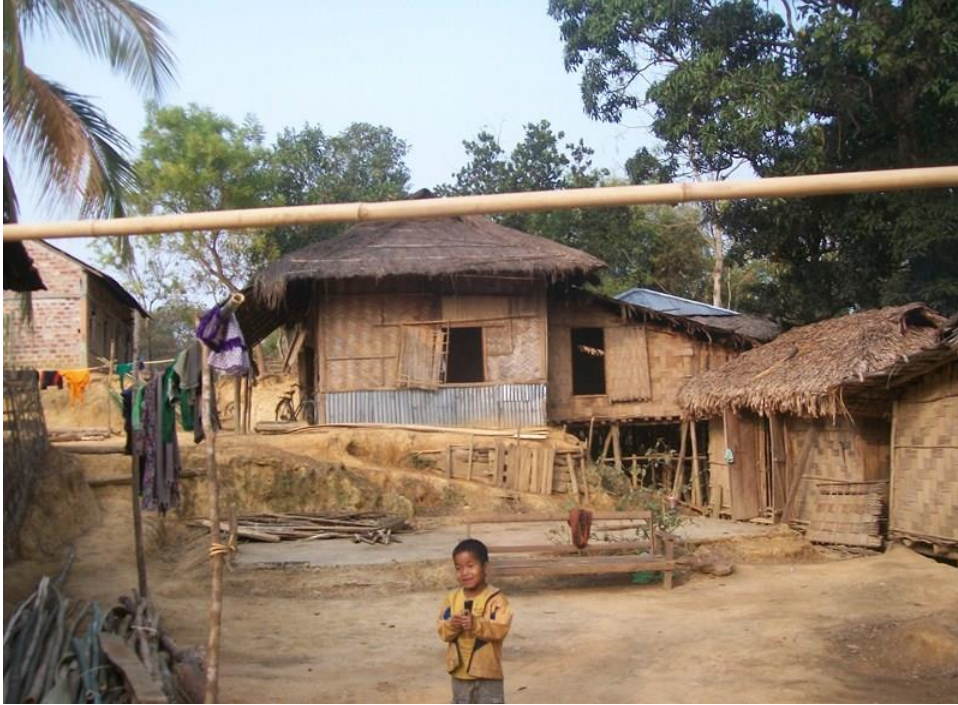
House Structure of Kuki Community in Nagathal
