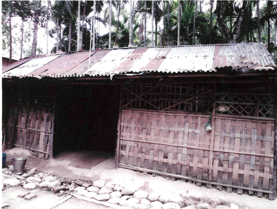
House of a day labourer which made up of tin and bamboo wall. Majority of the houses of Patni community are of the same type.
